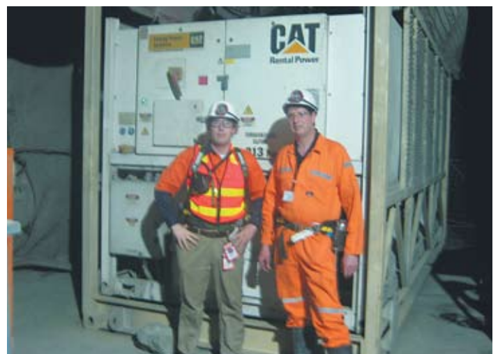
EPSA's CEO Phil Canning visits Stawell Gold Mine 1370 metres underground to see how well CAT Rental Power's temperature control is performing.
